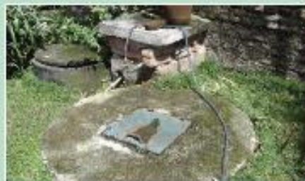
Groundwater recharge through dugwell
